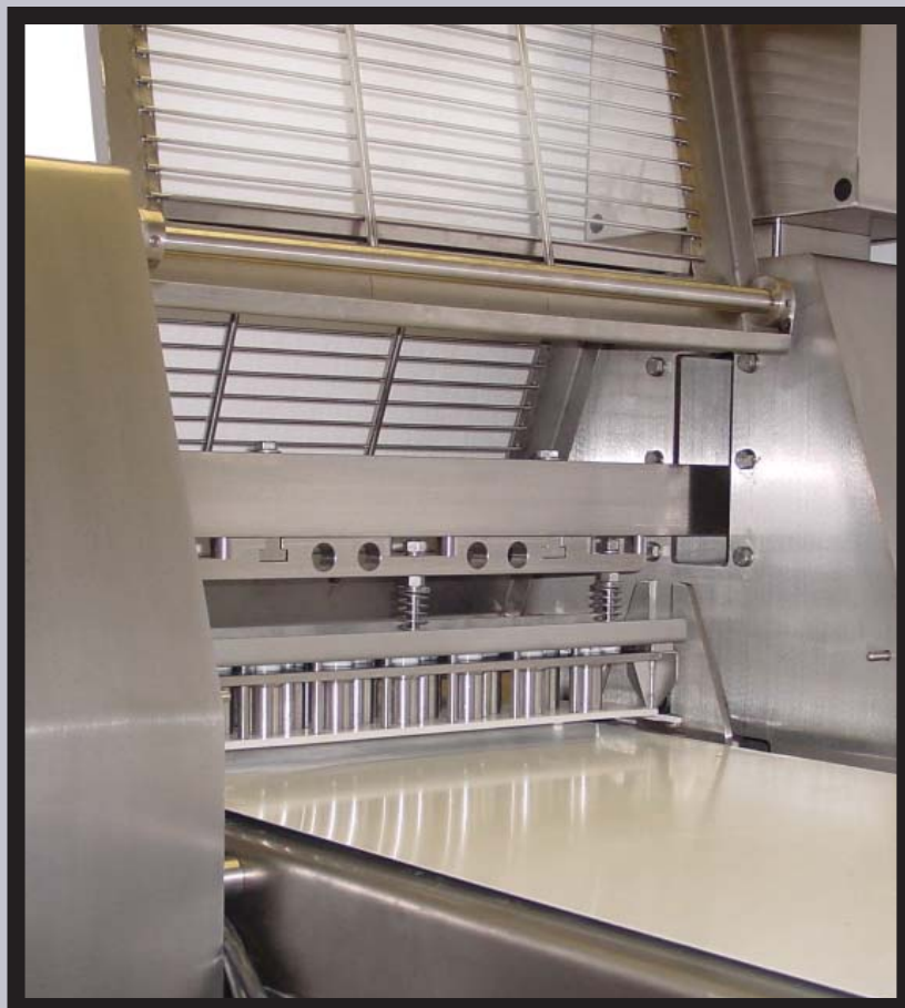
Stamping Die Installed in the Stamper
